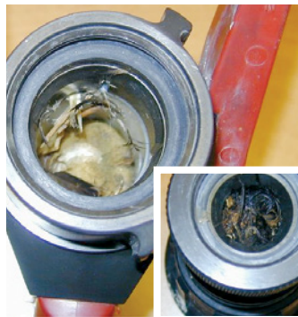
FDCs left vulnerable to debris, clogging the pipes
