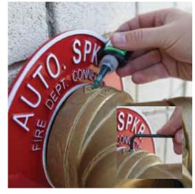
Clean drill holes of debris then place a small amount of remaining Permabond HM162 in hole and on set screws, then install set screws, securing firmly with a 5/32" Allen wrench.
