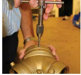
Tap threads in the hole/s using a 5/16-18 thread tap.
