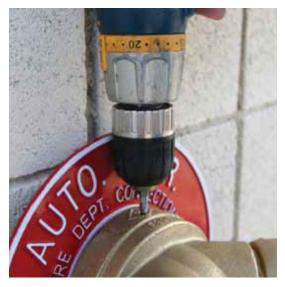
Use 1/4" drill bit to spot drill through the set screw hole/s in adapter and into pipe approximately 1/16" deep. **DO NOT OVERDRILL TOO DEEP AND PIERCE PIPE.**
