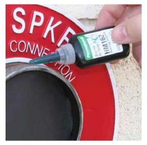
Apply Permabond HM162 to **BOTH** threads on adapter and threads on pipe. Coating should be thin, but needs to completely coat the threads.
