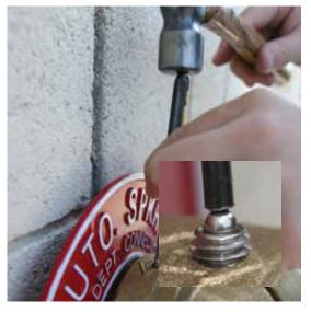
After set screws have been secured, insert a ball bearing slightly larger than the Allen socket hole into the screw head and use punch to hammer into place. Alternatively, fill the screw head with a permanent epoxy material.
