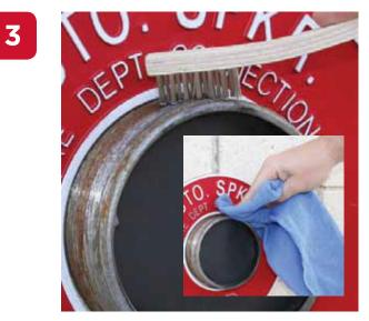
Clean pipe threads thoroughly with solvent, wire brush, and dry completely. **NO** grease or oil can be present on the pipe threads in order for adhesive to work properly.
