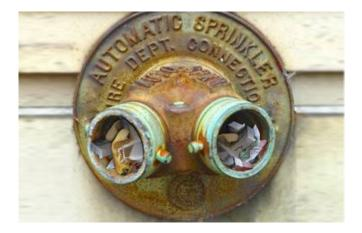
The FDC is the access point for a building's sprinkler system to receive supplemental water. Since most building owners are not aware of the importance of protecting FDC's, Chief Reid was looking for an effective, easy-to-implement solution that business owners could implement to protect and secure their FDC's from debris, damage and vandalism.
