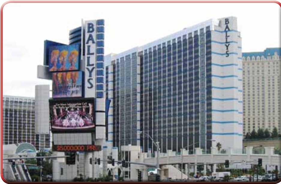
The former MGM Grand (now Bally's) as seen from Caesars Palace. On November 10, 1980, an electrical fire spread quickly and produced a massive fireball that blew out the main entrance. The burning material created toxic fumes and smoke, causing most of the 85 deaths. Faulty smoke dampers and an exemption to Fire Code are referenced as exacerbating this tragedy.
