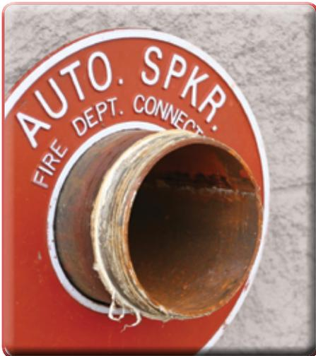
*Stolen FDC connections are being replaced with Storz connections and Knox StorzGuard locking caps in McKinney, TX*
