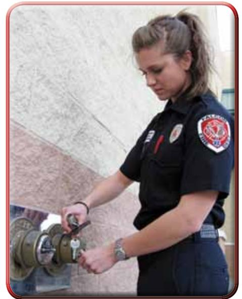
*Firefighter/EMT E. Frey installing a Knox FDC Plug.*
