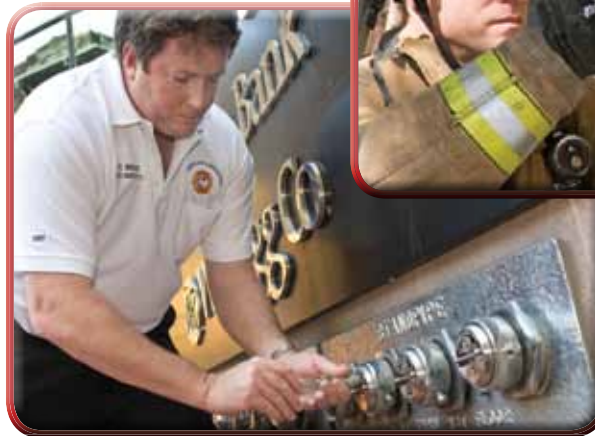
Inspector Paul Measles (left) installing Knox® FDC Plugs; Firefighter unlocking FDC plug (above)
